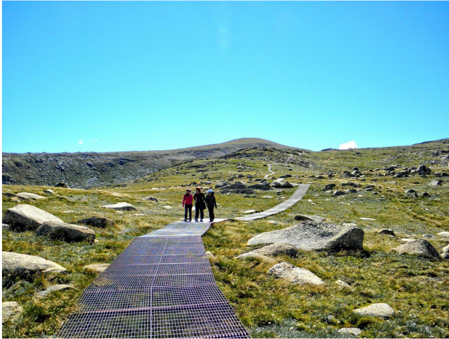
Photo 3.5-3. Steel-mesh walkway at Mt Kosciuszko, NSW. Photo by Paul Ma.
