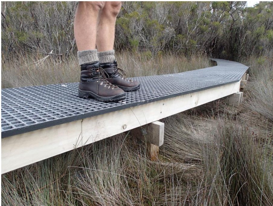
Photo 3.4. Walkway with 1m wide FRP walking surface at Melaleuca, SW Tas. Photo by Grant Dixon.
