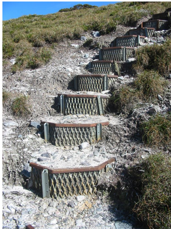
Photo 3.5-2. Steel-mesh step risers near Lake Cygnus, Western Arthur Range.
